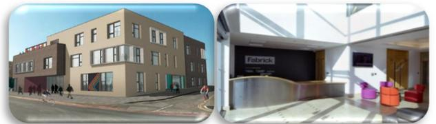
The central atrium is a significant feature of the building & not only assists in the cross ventilation strategy but also improves natural daylight penetration into the deeper plan offices.
